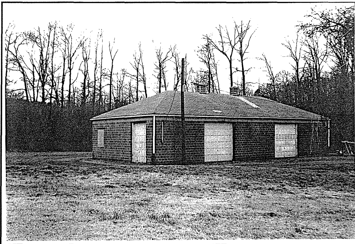
Photo ID: Building 062, South and East Facades, 2/97
