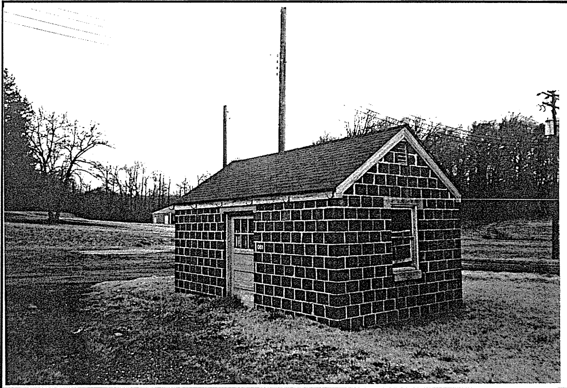
Photo ID: Building 061, South and East Facades, 2/97
