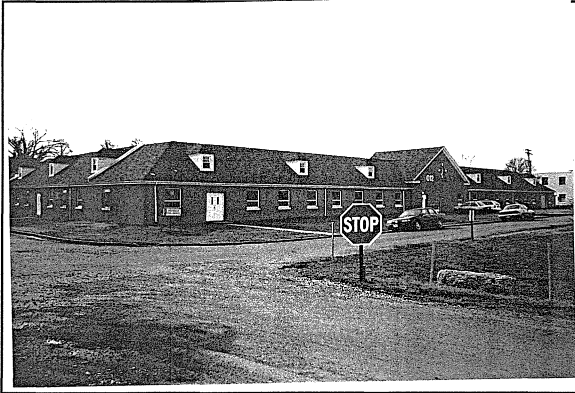
Photo ID: Building 012, East and North Facades, 2/97
