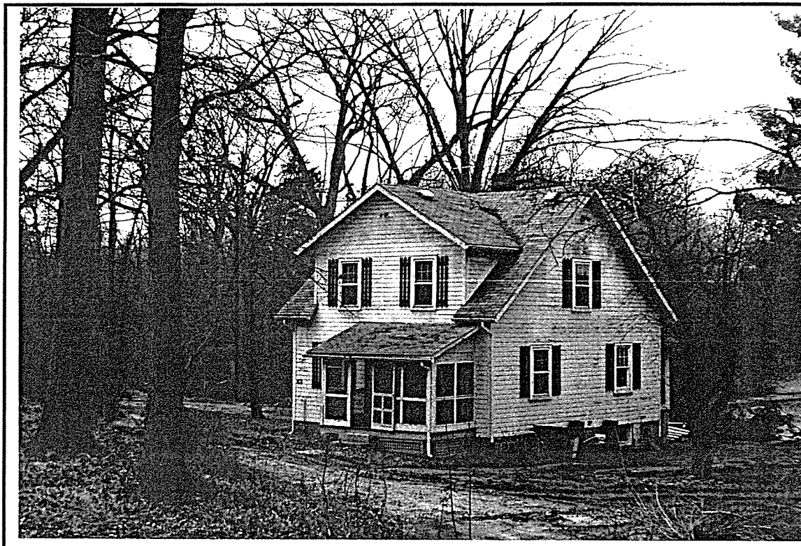
Photo ID: Building 016, North and East Facades, 2/97
