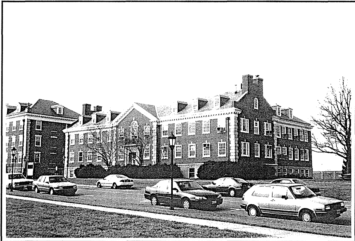
Photo ID: Building 004, East and North Facades, 2/97
