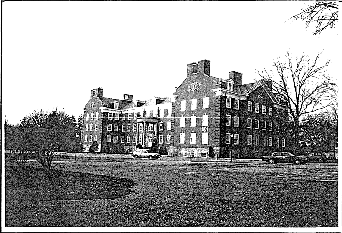
Photo ID: Building 001, East and North Facades, 2/97
