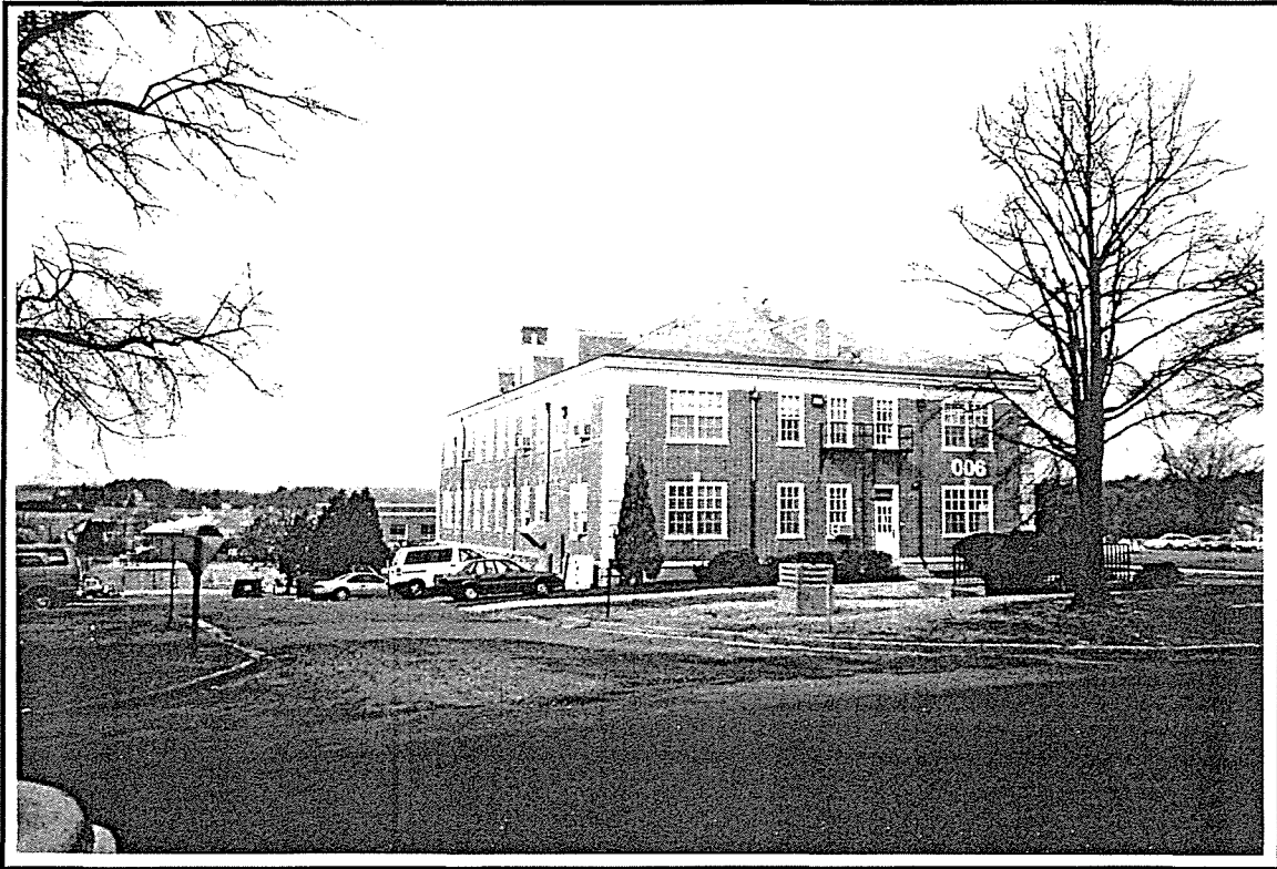
Photo ID: Building 006, South and East Facades, 2/97
