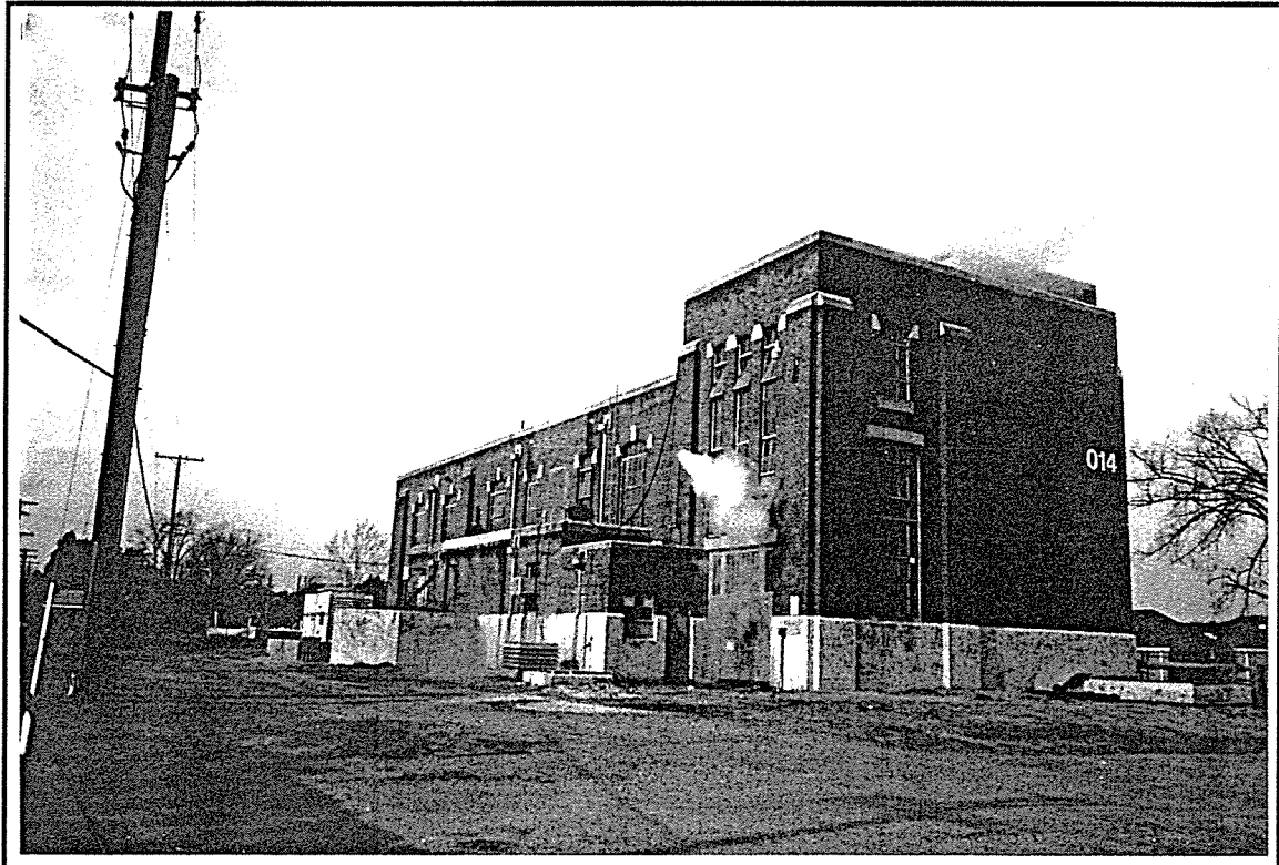
Photo ID: Building 014, East and South Facades, 2/97
