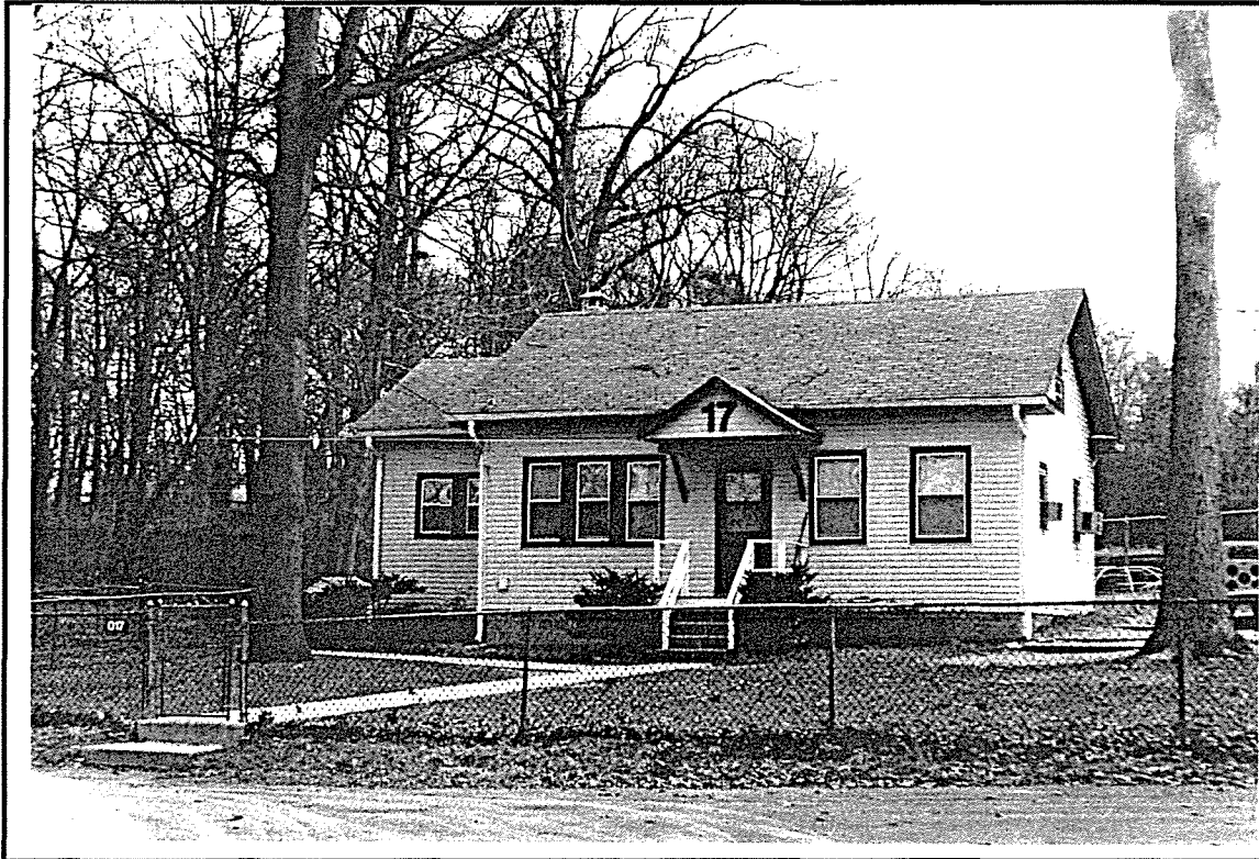
Photo ID: Building 017, West Facade
