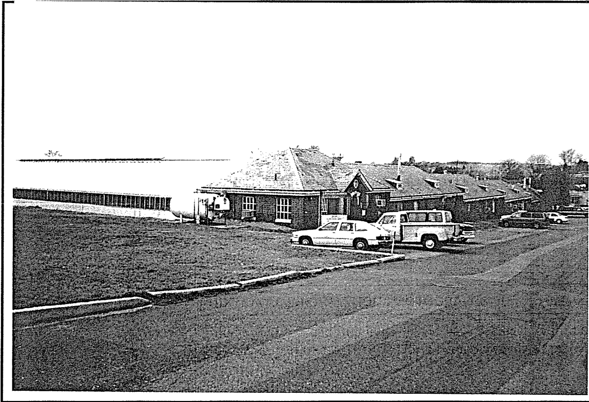
Photo ID: Building 010, East and North Facades, 2/97
