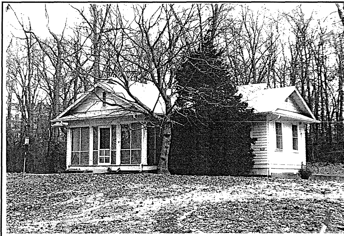
Photo ID: Building 018, South and West Facades, 2/97
