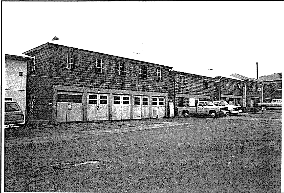
Photo ID: Building 029A, North Facade, 2/97
