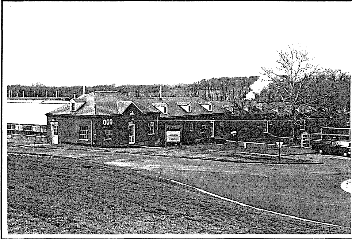
Photo ID: Building 009, East and North Facades, 2/97
