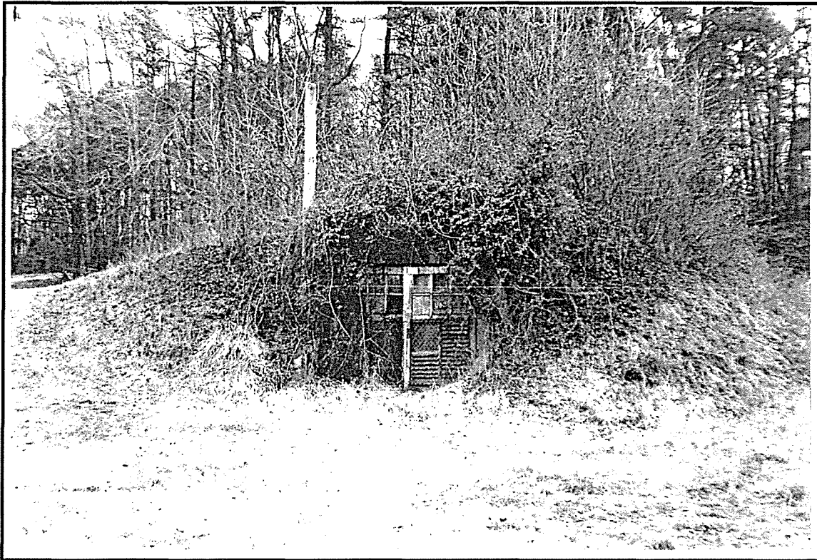
Photo ID: Building 063, North Facade, 2/97
