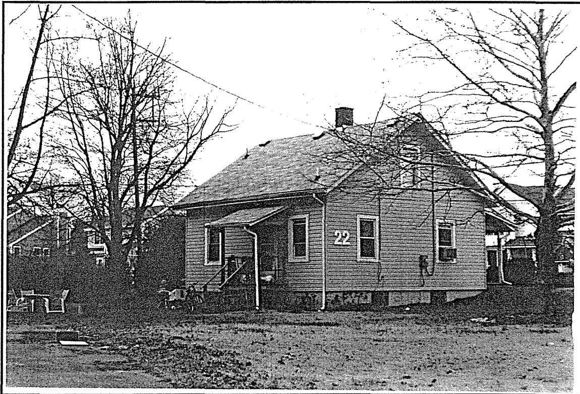
Photo ID: Building 022, South and East Facades, 2/97
