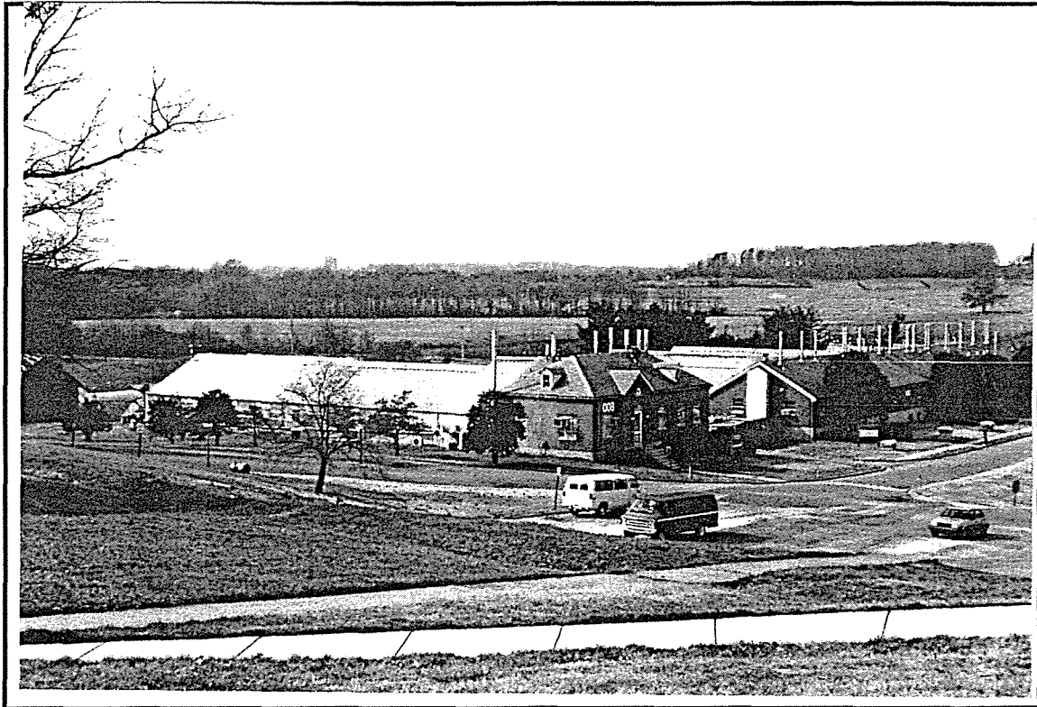
Photo ID: Building 008, East and North Facades, 2/97
